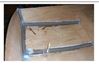
Figure 2 – Stitch N Glue joints with Peelply applied
