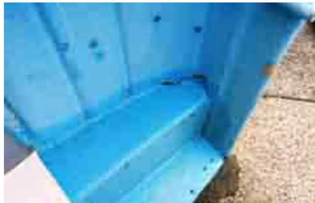
Figure three – Dinghy seat delamination.
