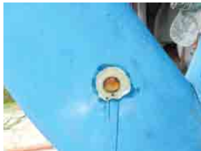
Figure eight – Vinylester FRP repair rework.
